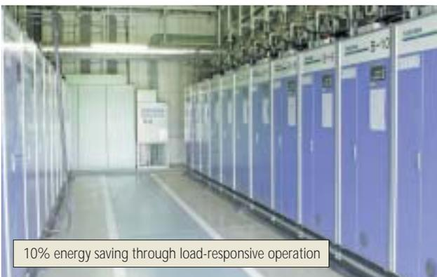
Fuel saved by controlling number of boilers in operation
